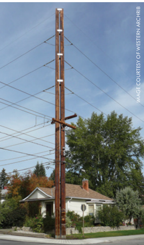
Two 107-foot poles are bolted together in this utility pole design.
