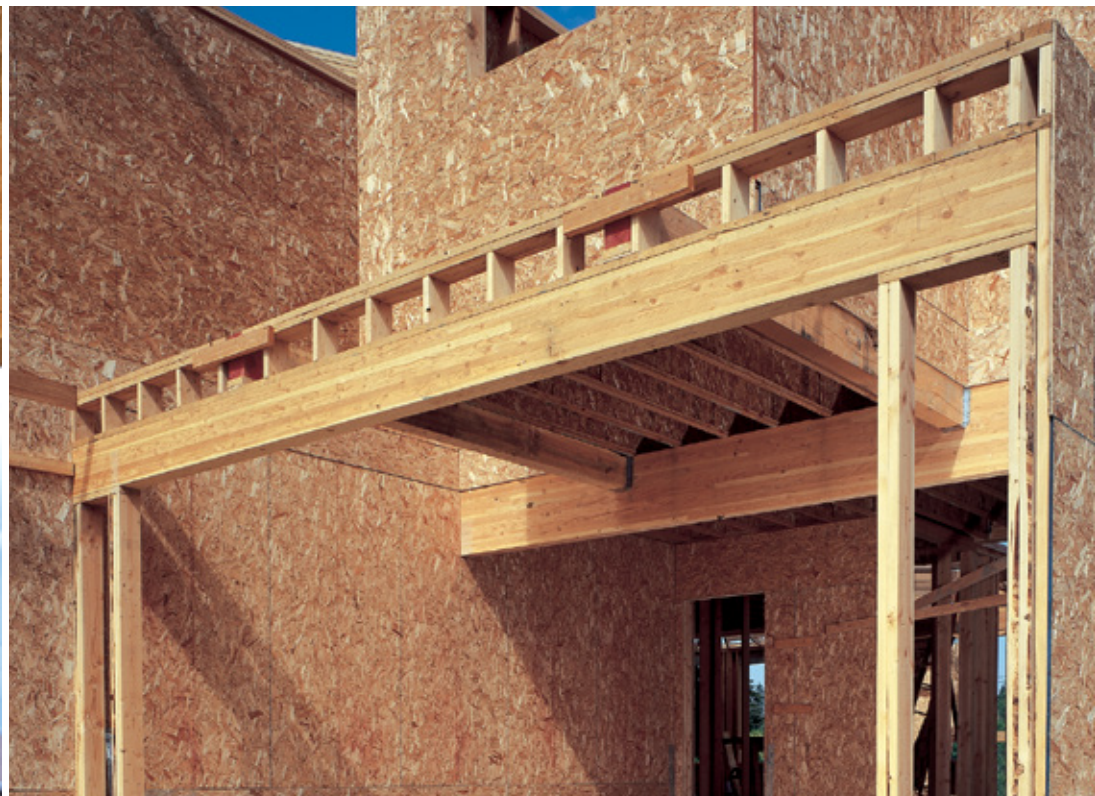
Glulam garage door header extends over adjacent narrow shear wall. (See Figure 4 for further details.)
