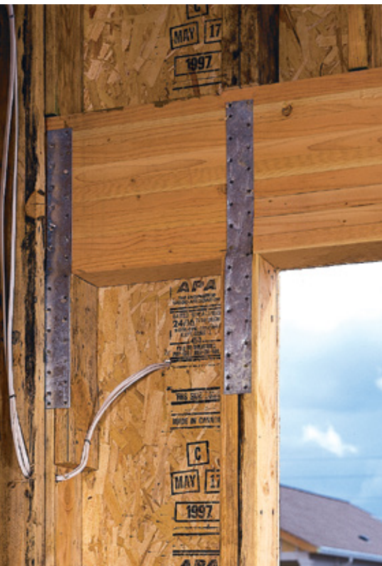
Glulam garage door header extends over adjacent narrow shear wall. (See Figure 4 for further details.)
