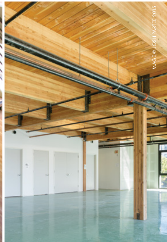
The One North office complex in Portland, Ore., uses glulam framing with tongue-and-groove cedar decking.
