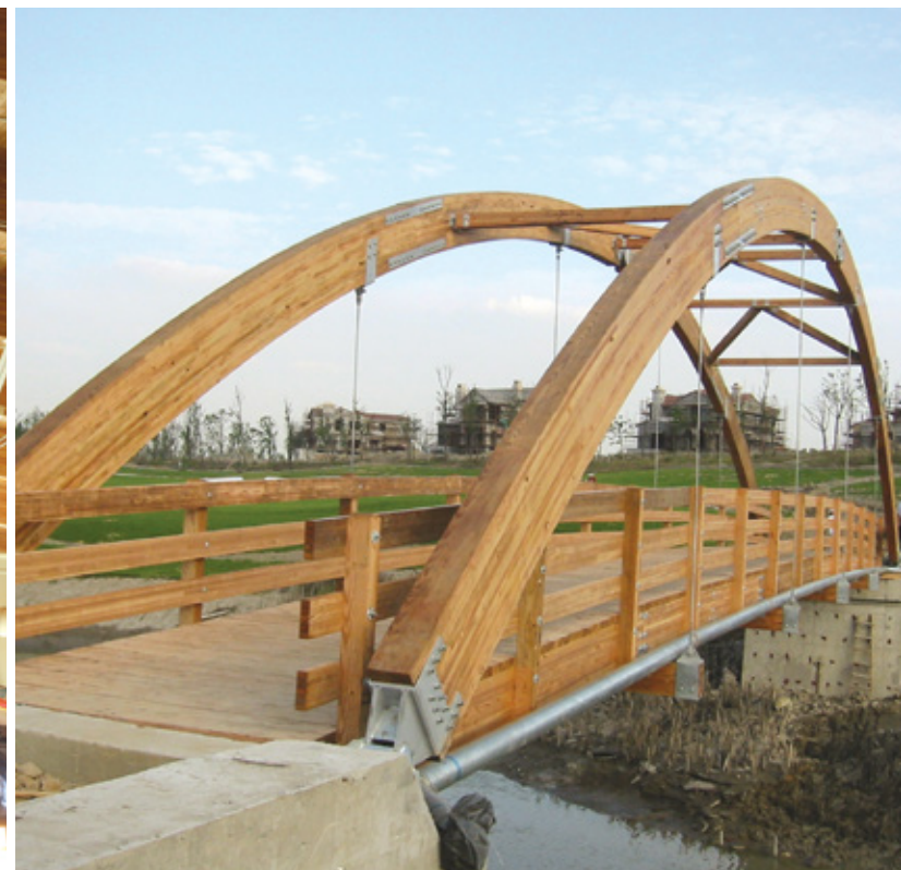
This glulam bridge connects the Sheshan Golf Course with a nearby luxury residential community, providing both style and functionality.
