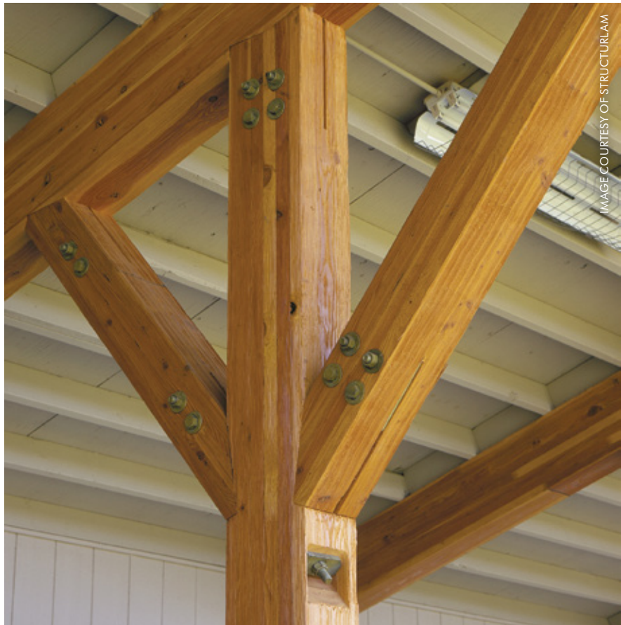
These glulam members use notches and hidden connectors, resulting in a clean, uncluttered design.
