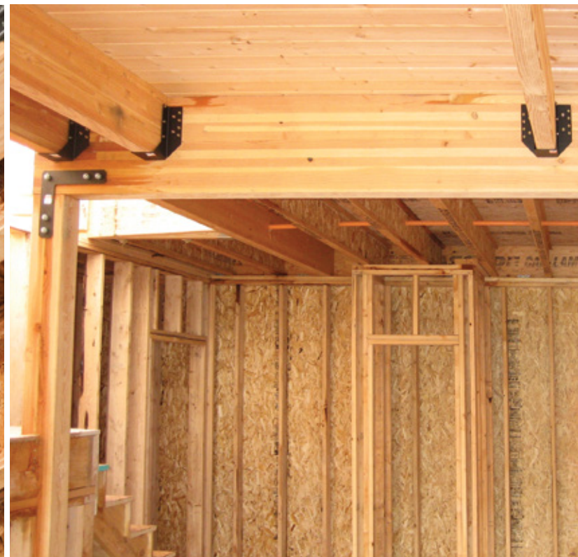
Glulam columns and headers provide primary support in this condominium construction.
