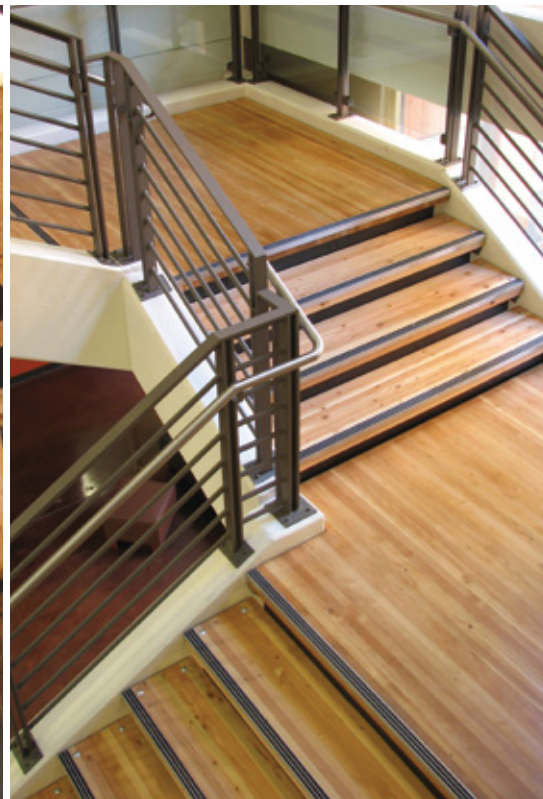
Durable glulam forms a stair tread.
