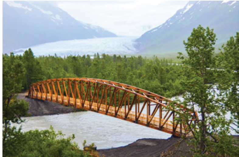
The Placer River Trail Bridge in Alaska uses glulam spans.
