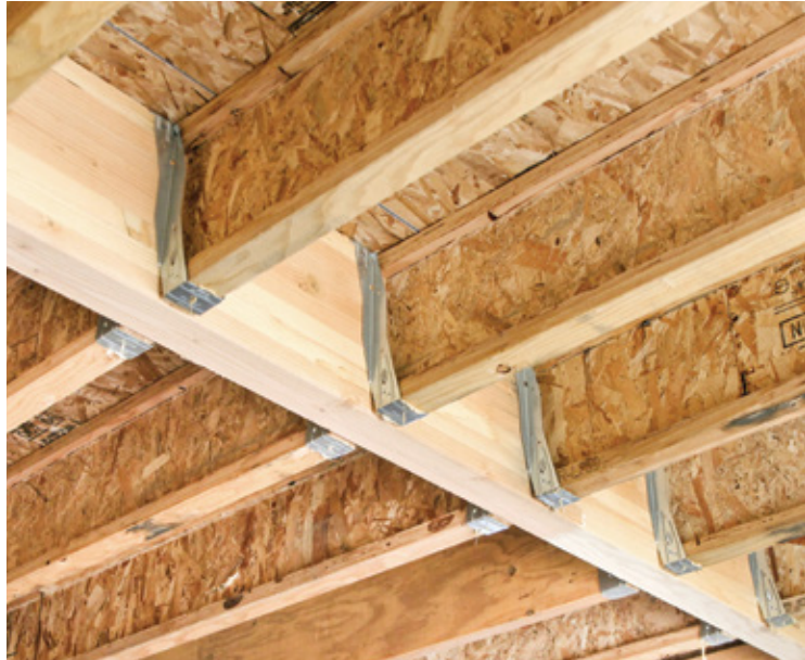
I-joist compatible (IJC) glulam beams are supplied in depths of 9-1/2, 11-7/8, 14 and 16 inches.
