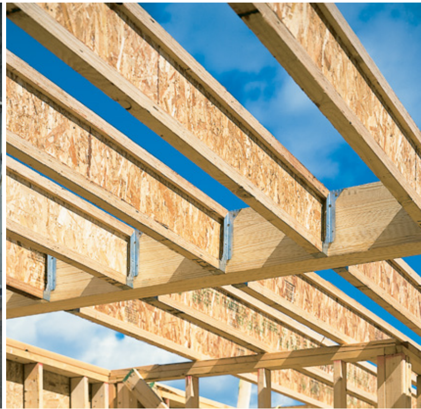
I-joint compatible glulam beams are used for a range of framing needs in residential buildings.
